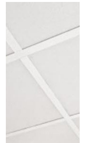
Suspended Ceiling Grid
